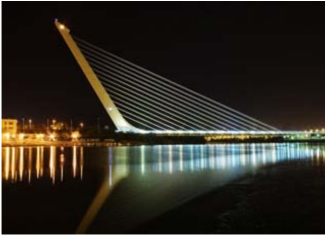
Figure 3.2. Alamillo Bridge, Seville
